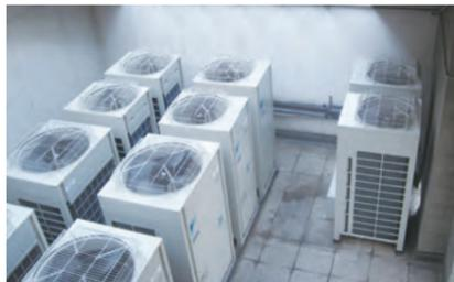
The original VRV units that ran on R22 were replaced with VRV III-Q units running on R410A.
