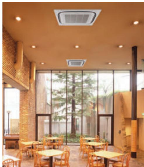
**Airflow pattern is selectable to match room shape and installation location**
