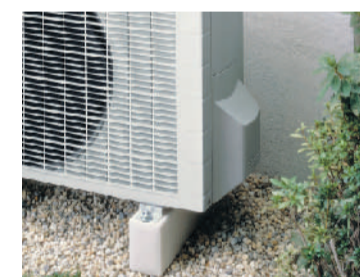
Piping connections for the outdoor unit are covered to make them less conspicuous.
